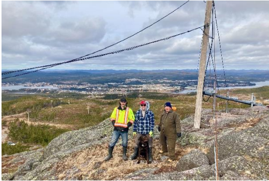
Photo 5. Members repairing our Communications Building on the Tolt following wind damage.
