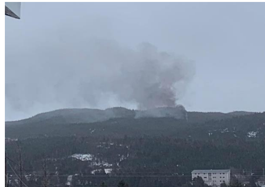
Photo 2. Structure Fire behind Dunphy's Road.
