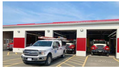
Photo 5. Paging System installation completion.
