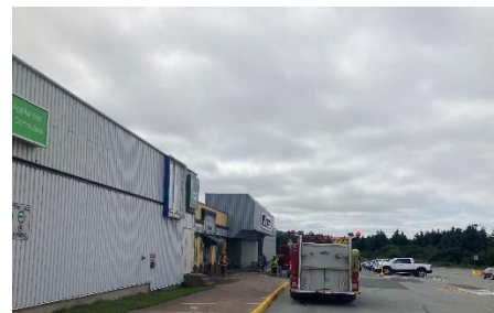
Photo 12. Fire Alarm at Peninsula Mall.
